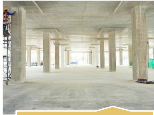
Flat Slab Flat Plate, Flat Slab
