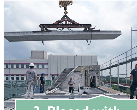
3. Placed with Cranes
